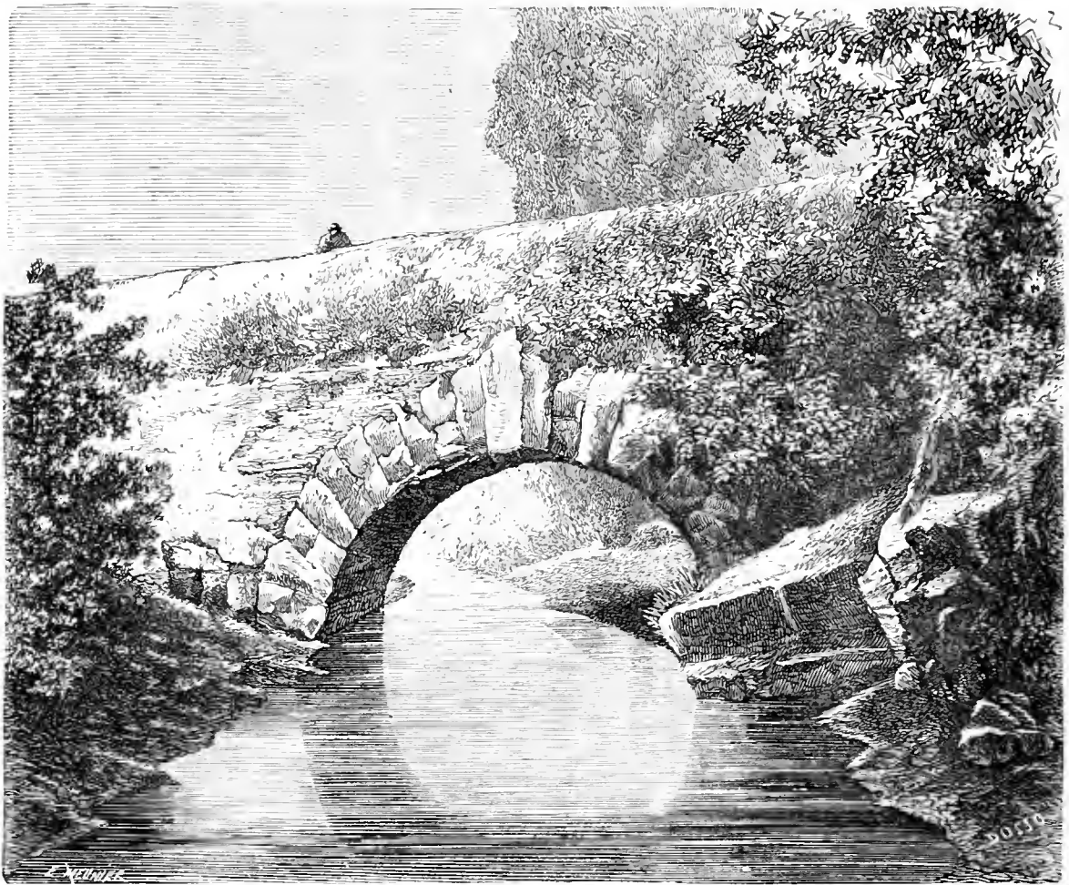
Roman Bridge over the Ostian Road.
